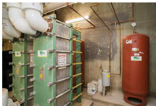
Taco plate-and-frame heat exchangers were selected for the heating and DHW loop in order to meet the high pressure demands of the system.
